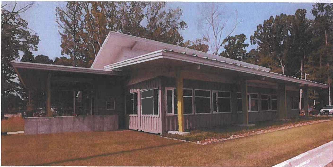
The southwest Little Rock, Ark., headquarters of Hugg & Hall is built out of Hugg & Hall Mobile Storage's own product ... shipping containers.
